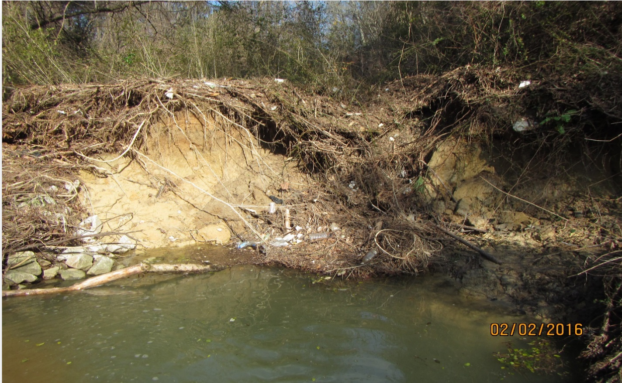
Figure 4: Bank erosion on Terrell Creek
